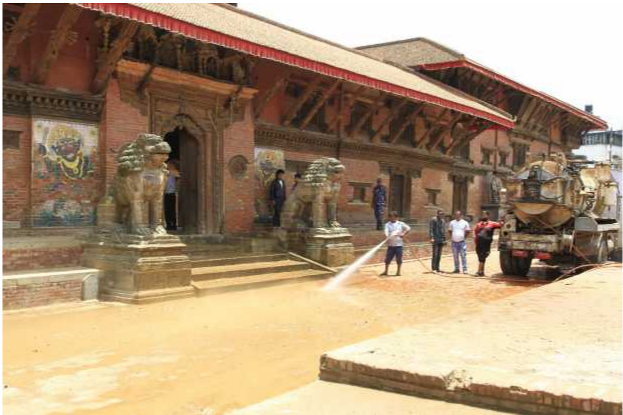
Final cleaning at Patan Durbar Square
