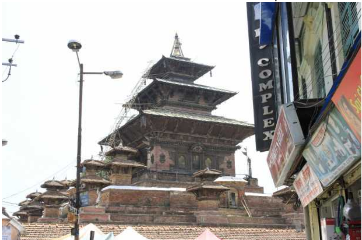
Maintenance of minor damage in the temples started
