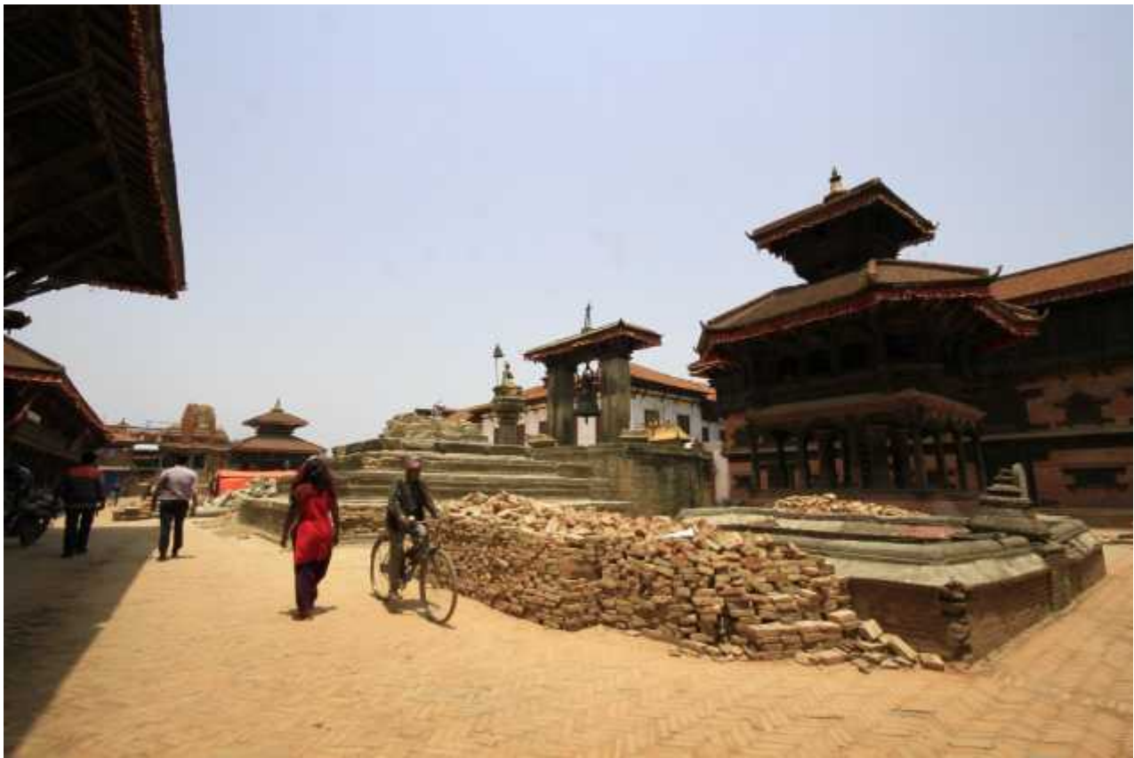
Clearing of rubbles at Bhaktapur Durbar Square is in final stage
