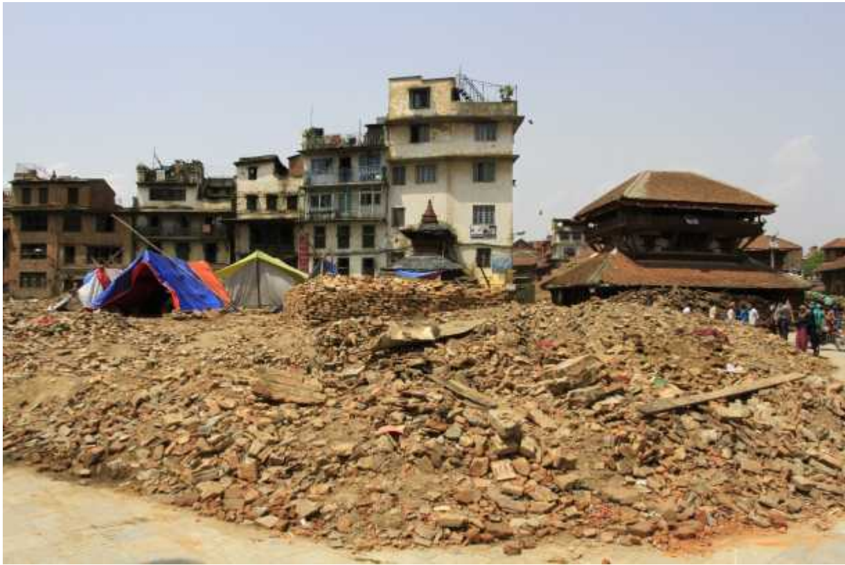
Debris from Kasthanadap which is completely destroyed
