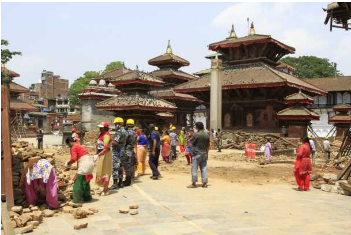
Cleaning of the rubbles in Kathmandu Durbar Square is going on
